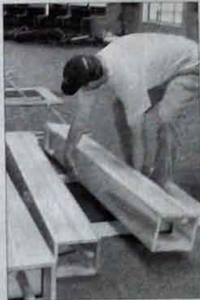
Two services this Sunday will go ahead as normal in the Langley Canadian Reformed Church sanctuary, despite the presence of scaffolding around the pulpit, explained church organist Frank Ezinga (far left). The church has spent years planning and renovating (left) the worship space to accommodate the new pipe organ which arrived in pieces (above) Tuesday.
